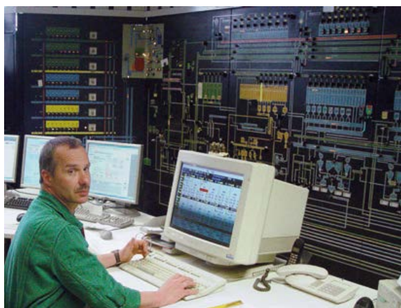
Figure 2: The central control room of the RKW plant where process information is analyzed.
